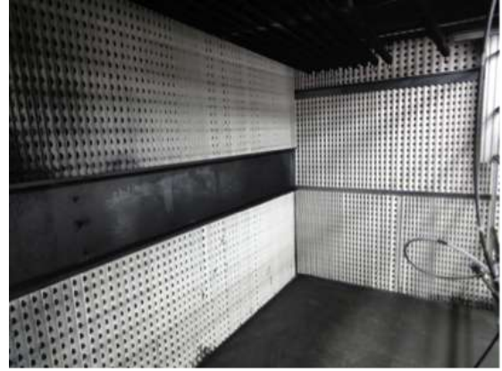
Figure 7.6: Filters and hanging rails for cathode boards
