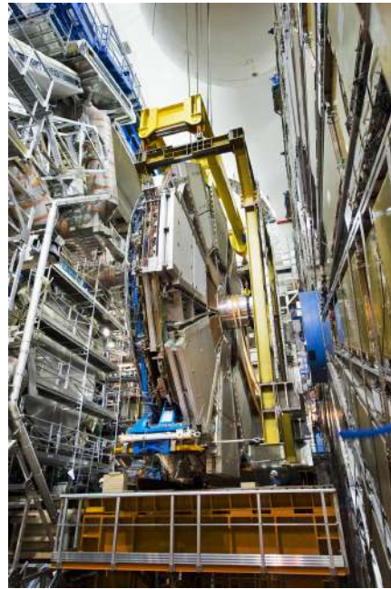
(d) Positioning of the SW on the HF-truck. The truck connects to the ATLAS barrel rail system.
