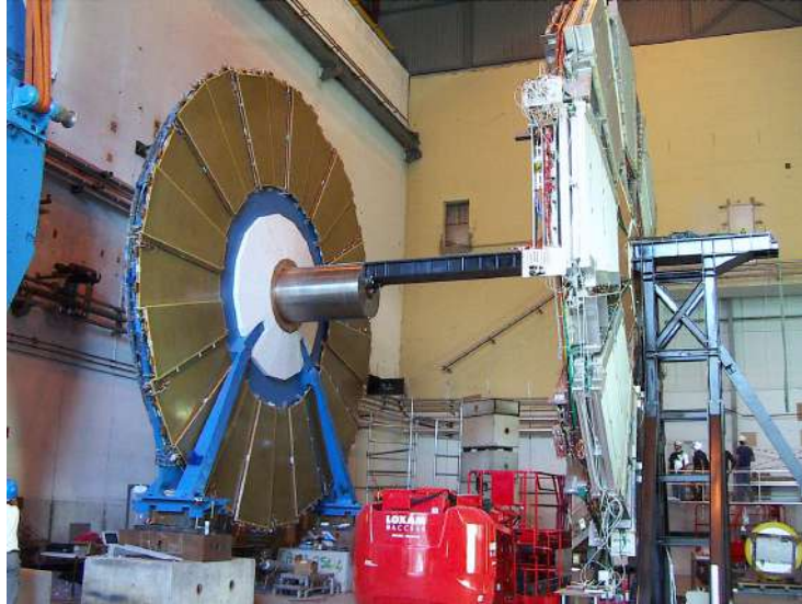
Figure 9.5: Integration of the detector wheel with the JD shielding in 2007. The wheel is transferred from the support structure (right) to the plug of the JD shielding (left) via a temporary rail (middle). The procedure used for the integration of the new detector wheels with the JD shieldings will be similar but the support structure and rail will differ.
