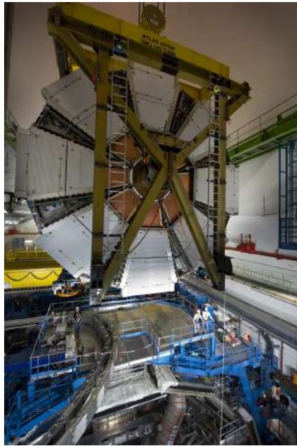
(c) Arrival in the experimental cavern. At the bottom, part of the ATLAS detector is visible.
